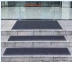
镂空设计，便于疏水 Easy to hydrophobic
